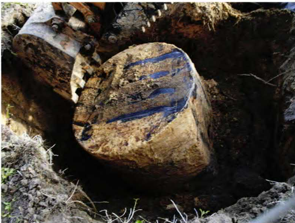
Picture 2: UST 527LaurelBB removal in progress.
